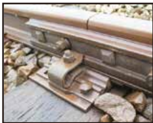
Installed with ordinary nuts
