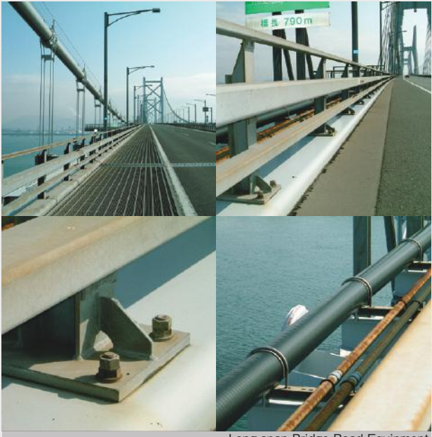
Long-span Bridge Road Equipment
