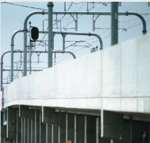
Steel Column Flange Stop
