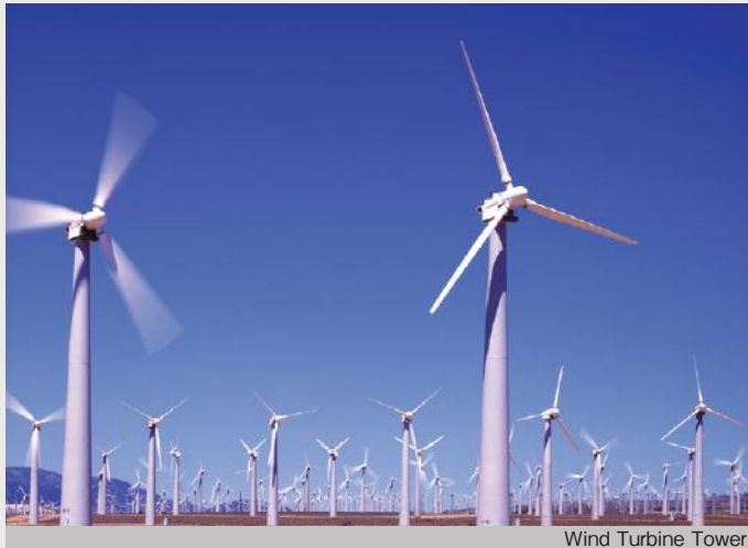
Wind Turbine Tower
