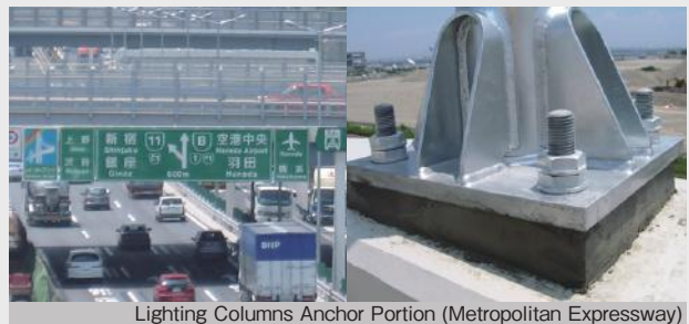
Lighting Columns Anchor Portion (Metropolitan Expressway)
